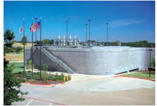
Control system design and programming for 32.5-mgd WTF hydraulic expansion using Allen-Bradley and Modicon PLCs, iFIX SCADA and Historian software.
