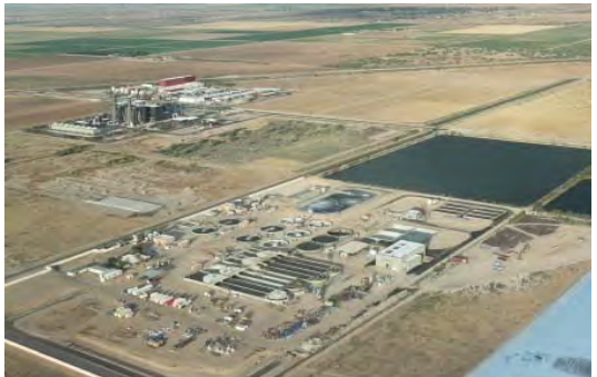
This large scale plant upgrade included the addition of 17 new (for a total of 26) PLCs as well as a completely new Wonderware system, including an enterprise-class Historian.
