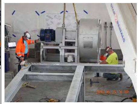
Photo #34 Area 50 Biosolids (looking northeast) on Friday, June 29 th . Hoffman is utilizing a mobile crane to help pipefitters for University Mechanical install a hot gas fan.
