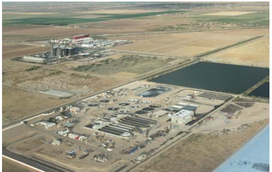
This large scale plant upgrade included the addition of 17 new (for a total of 26) PLCs as well as a completely new Wonderware system, including an enterprise-class Historian.
