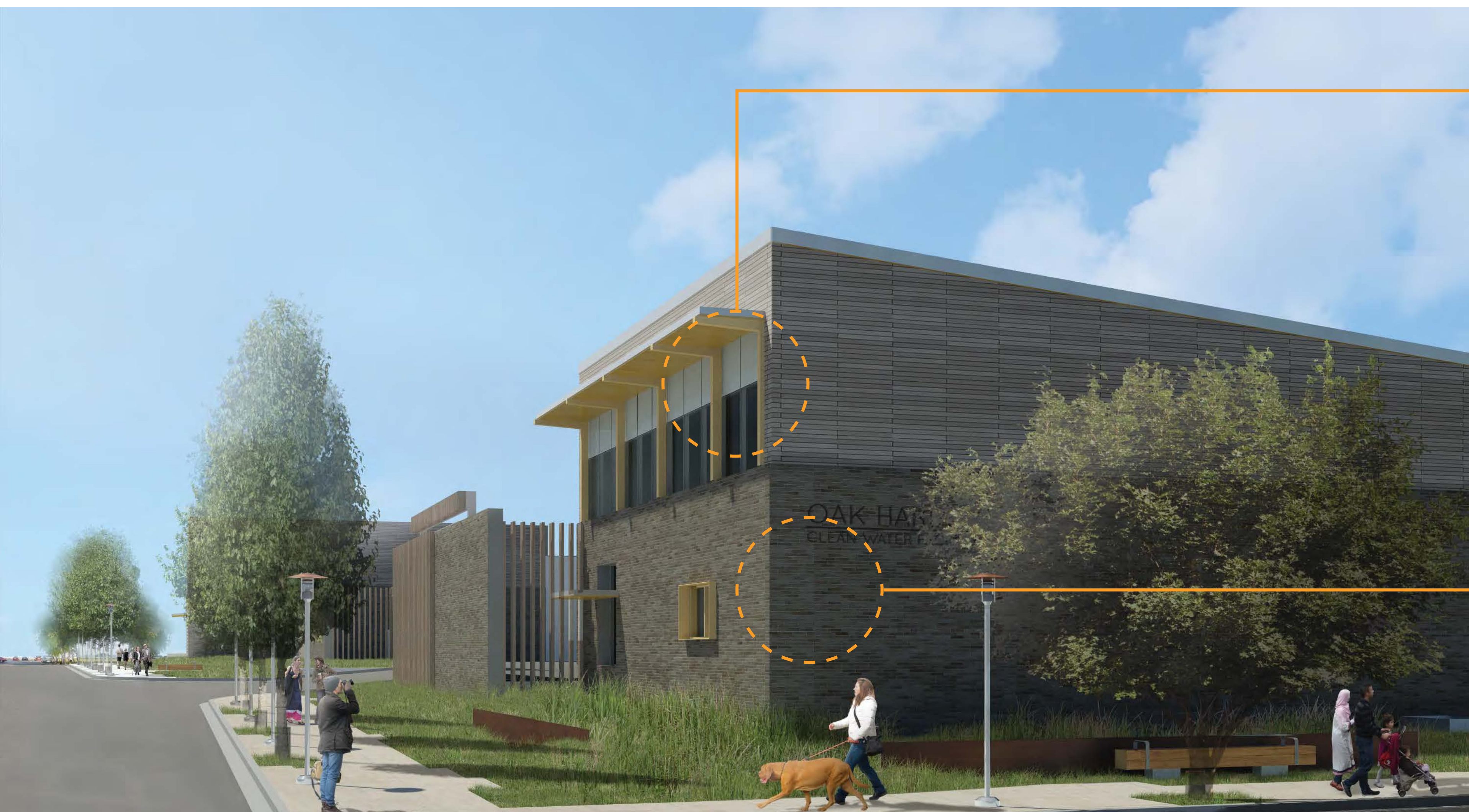
Headworks Building - View from Northeast
