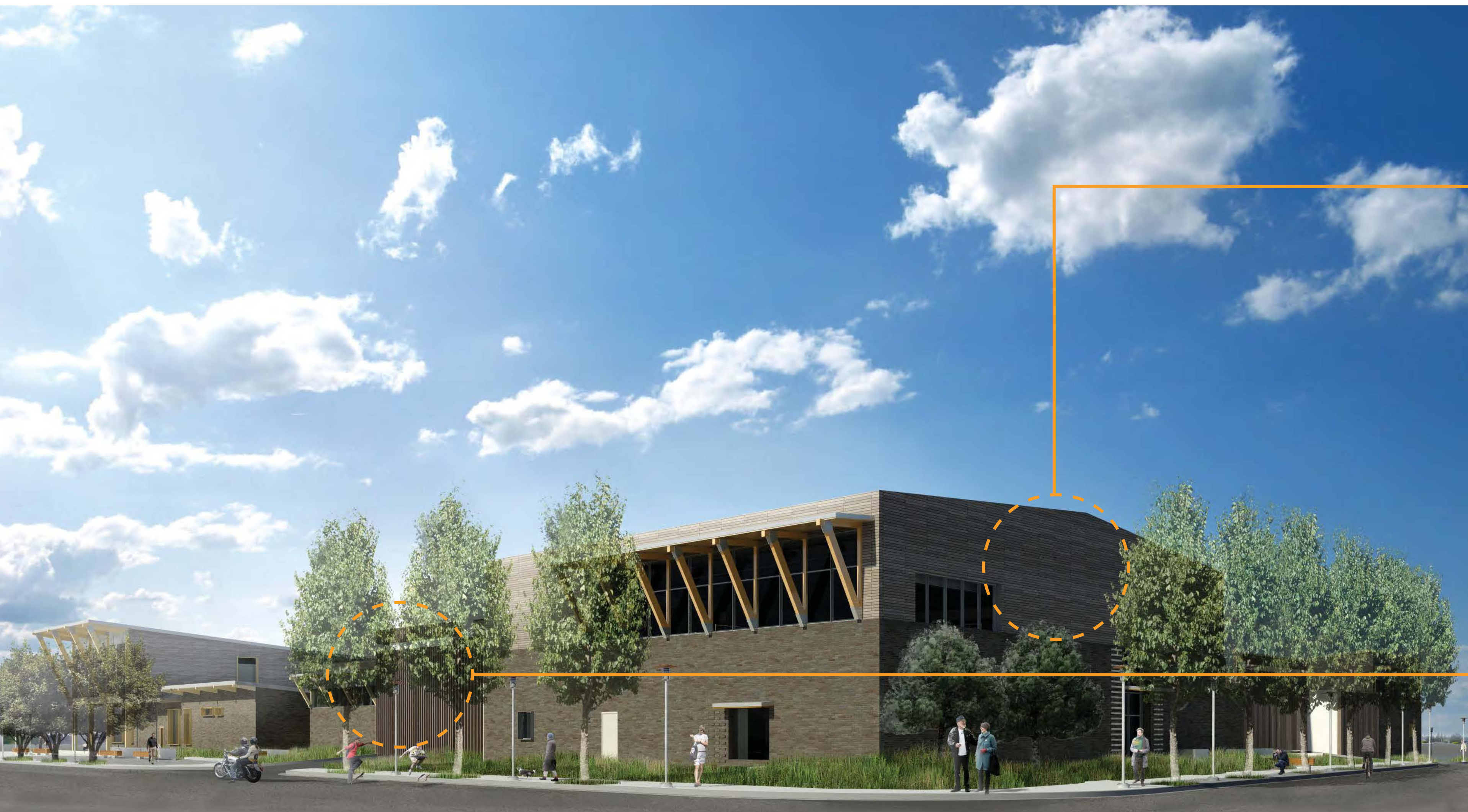
Solids Building - View from Southeast
