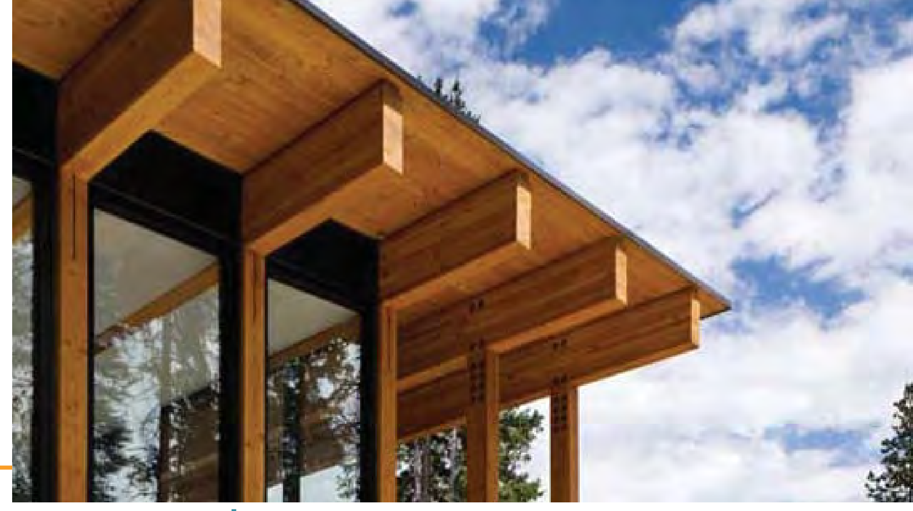
Heavy Timber Framing
