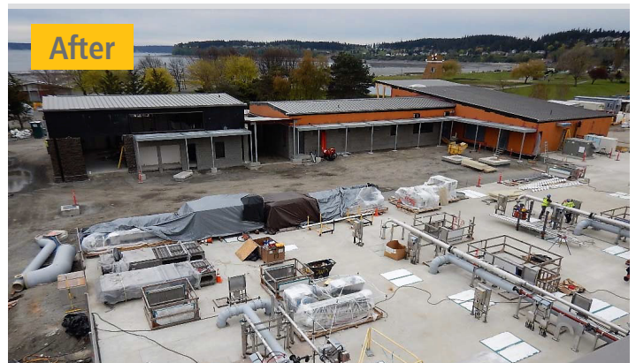
Look how far we've come! Before and after view of the maintenance and administration buildings at the new Oak Harbor Clean Water Facility.
