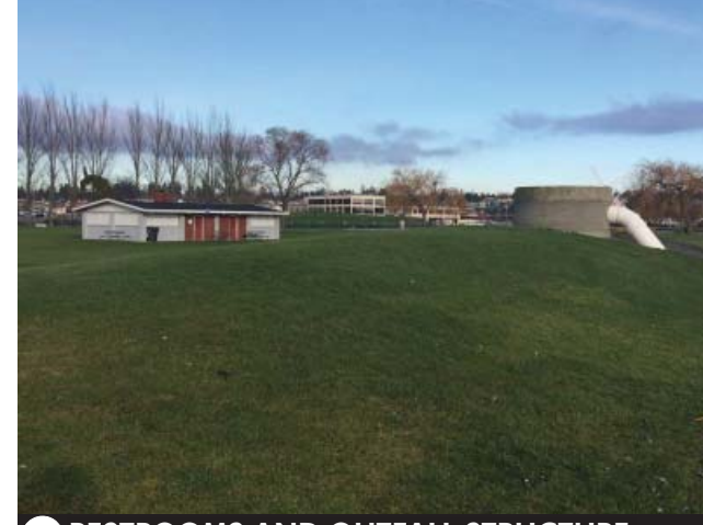
7 RESTROOMS AND OUTFALL STRUCTURE
