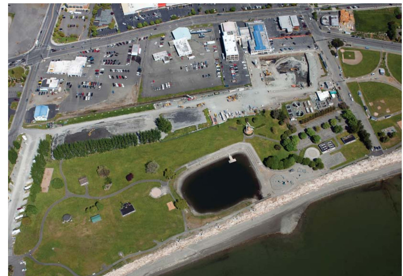
CWF Construction Footprint, May 2016
