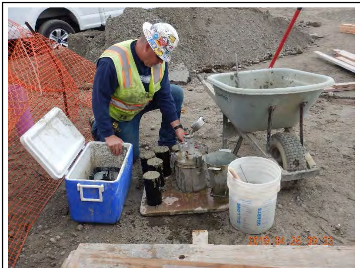
A special inspector for GeoTest, Zack Click, is measuring air content in a sample of concrete.
