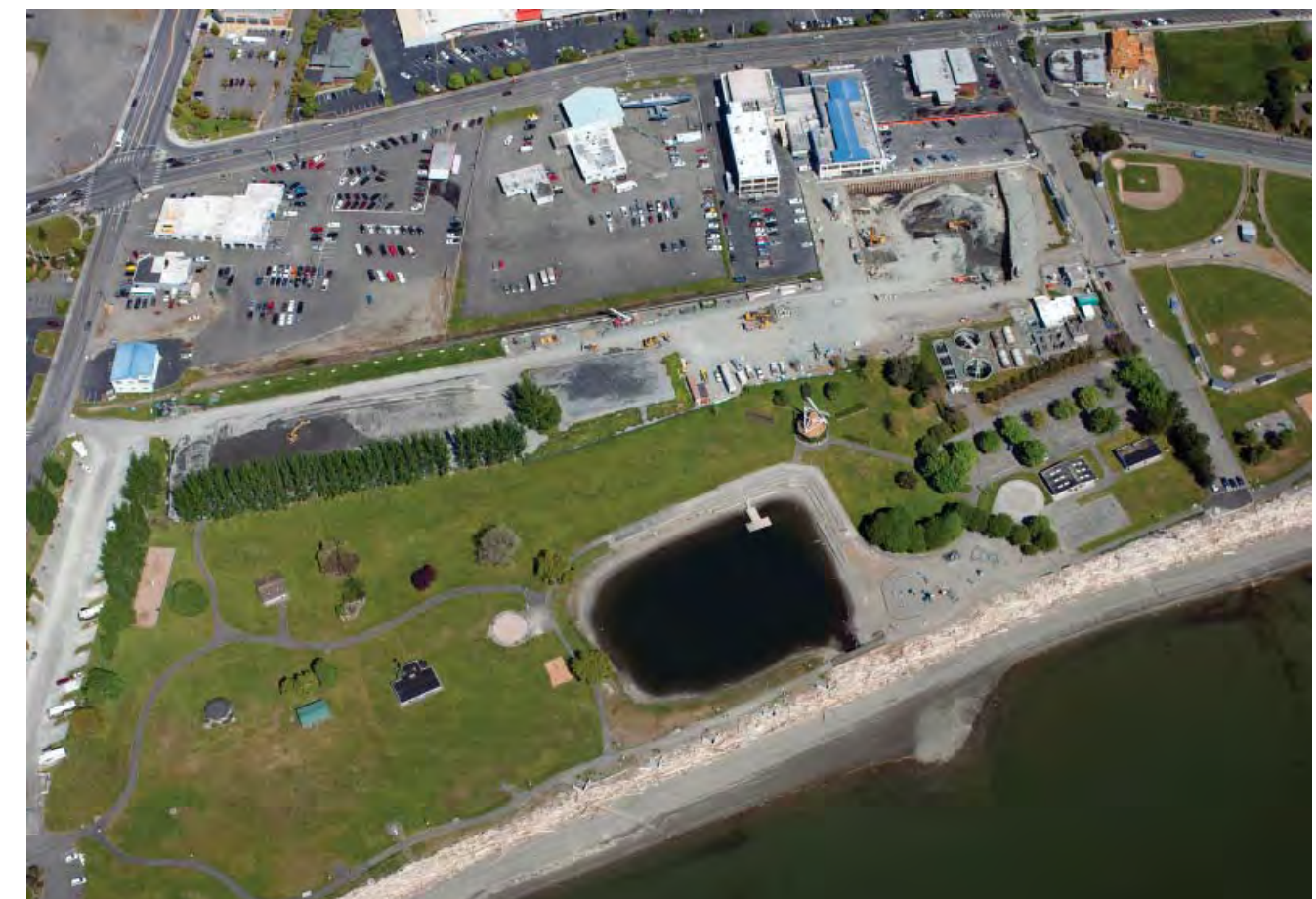
CWF Construction Footprint, May 2016
