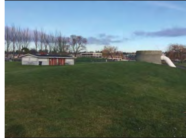
7 RESTROOMS AND OUTFALL STRUCTURE
