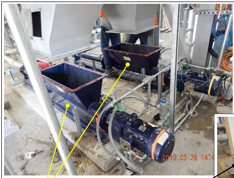
Dryer Feed Pumps
