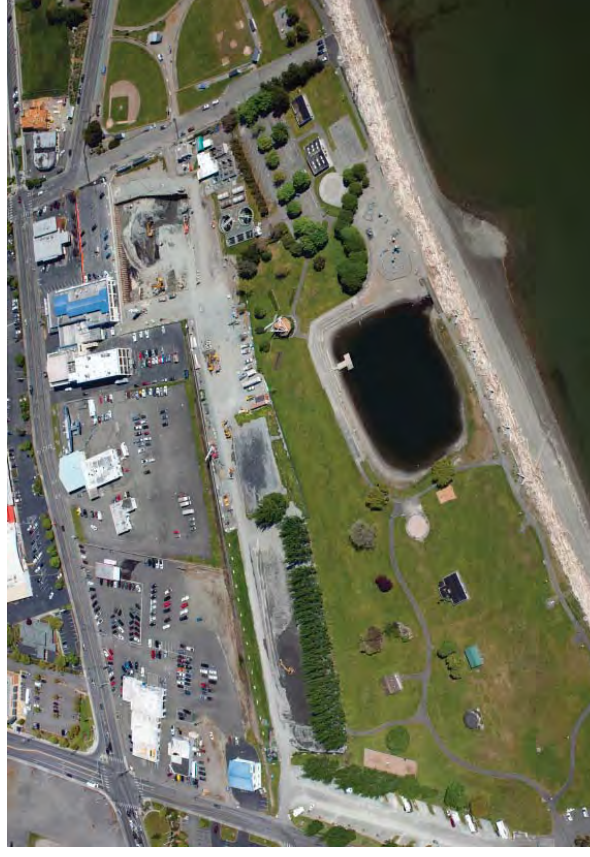
CFW Construction Footprint, May 2016
