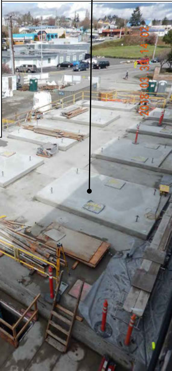
Removable Concrete Cover (typical)
