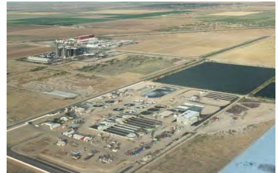
This large scale plant upgrade included the addition of 17 new (for a total of 26) PLCs as well as a completely new Wonderware system, including an enterprise-class Historian.
