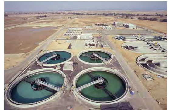
Carollo Engineers designed a system that would meet Roseville's need for "unattended operations" at the Pleasant Grove facility.
